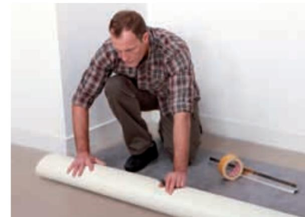
N.B. Only material cut into strips which include the manufactured sheet edges are suitable for utilising for fill-in sections. This factory edge must be reversed and abutted to the previous sheet installed. Do not install strips that do not have a manufactured edge, as there is a potential risk of shading.
